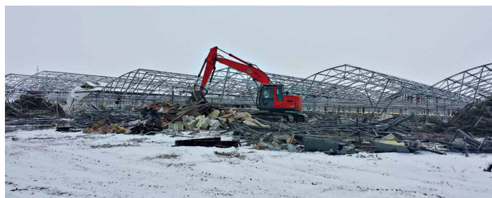
Dismantling and demolition work of above-ground facilities during Phase 1.
