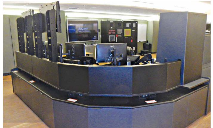
To prepare for the expansion start-up, we upgraded a number of existing PE1 plant facilities including the control room.
