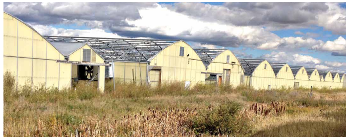
Before: The above-ground facilities included three greenhouses, a warehouse and some associated smaller buildings.
